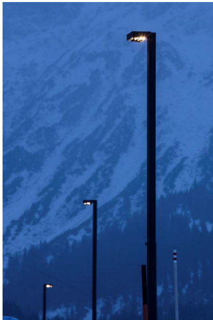
Fig. 4: The luminaires can be configured with 6 to 34 LED points, each with approx. 2 W.
