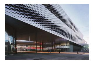
**Caption 1**: Above the glazed ground floor of the new trade fair building two further hall structures stand up, featuring an impressive facade consisting of interweaving aluminium bands.
