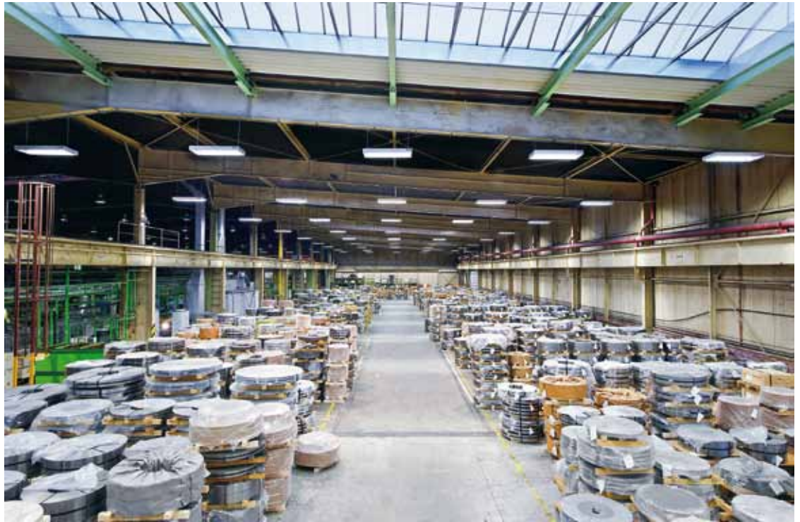
B3 | Zumtobel's Valuea high-bay luminaires are fitted with state-of-the-art fluorescent lamps and high-performance reflectors, ensuring a high-quality lighting effect.
